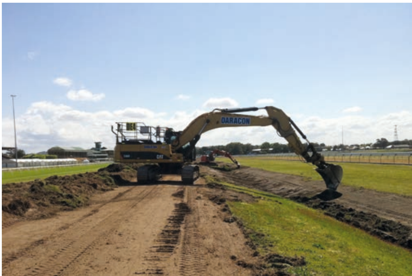
Project Commencement – Stripping Turf from the B-Grass Swale Drain, October 2014
