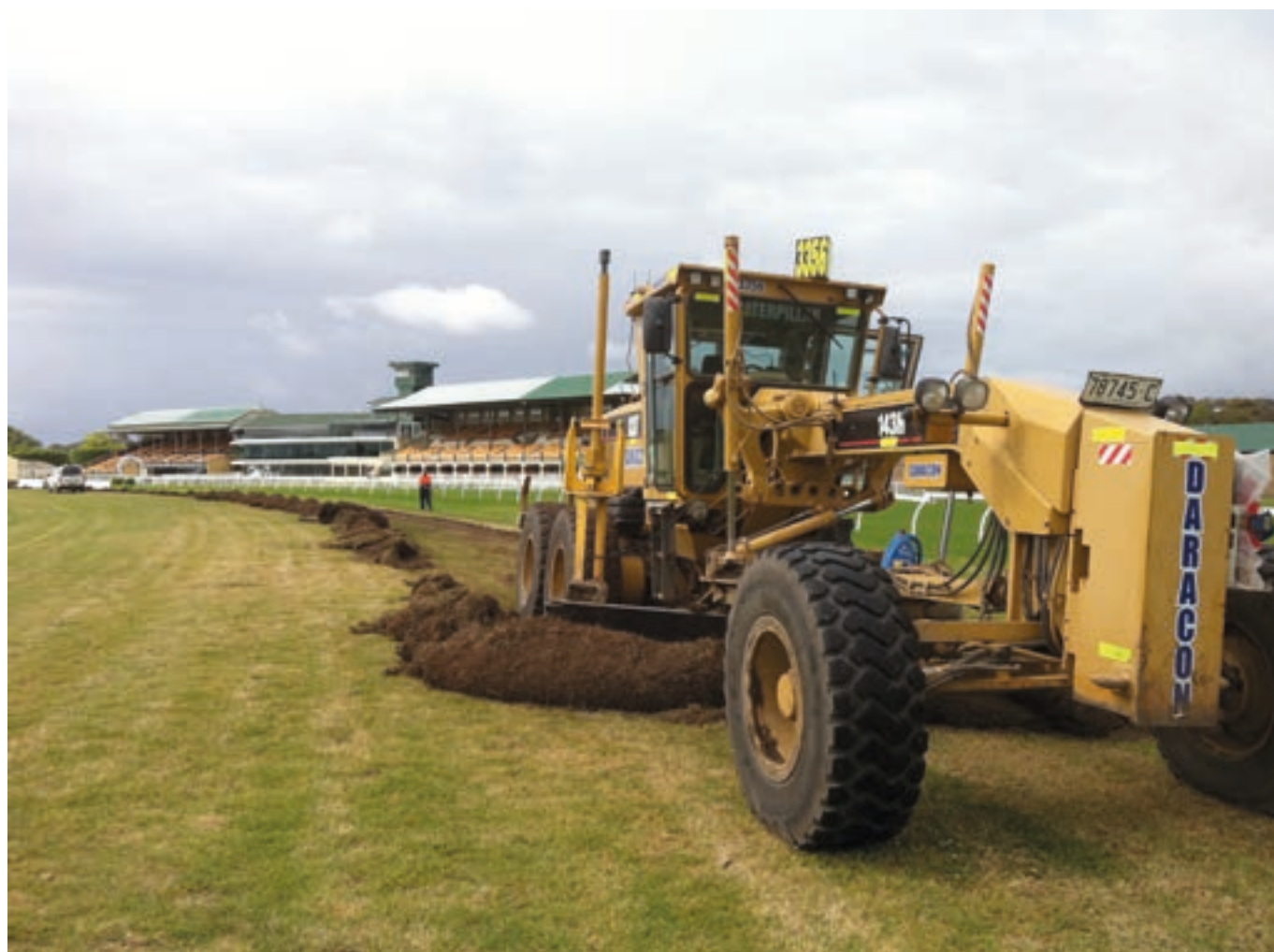
Project Commencement – Stripping Turf from the B-Grass Training Track, October 2014
