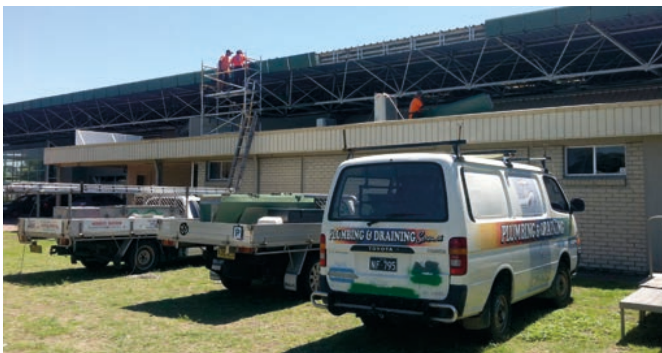
Betting Ring Box Gutter Replacement
