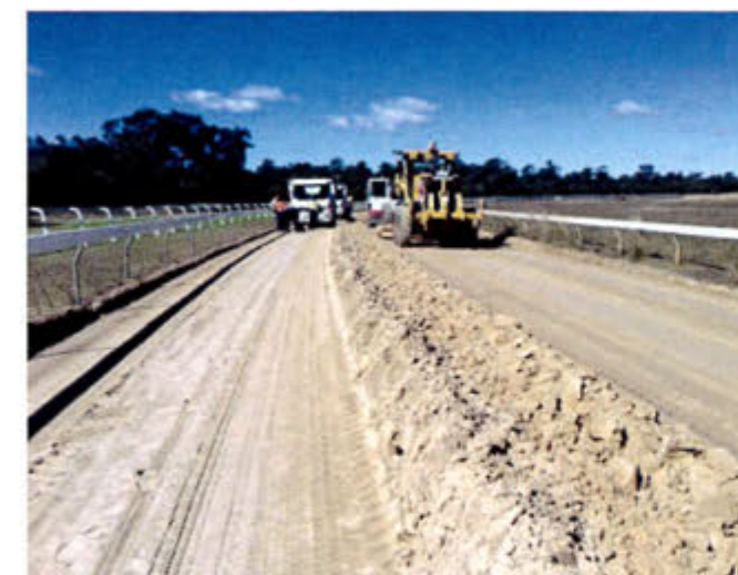
Storm Damaged Sand Track Repairs
